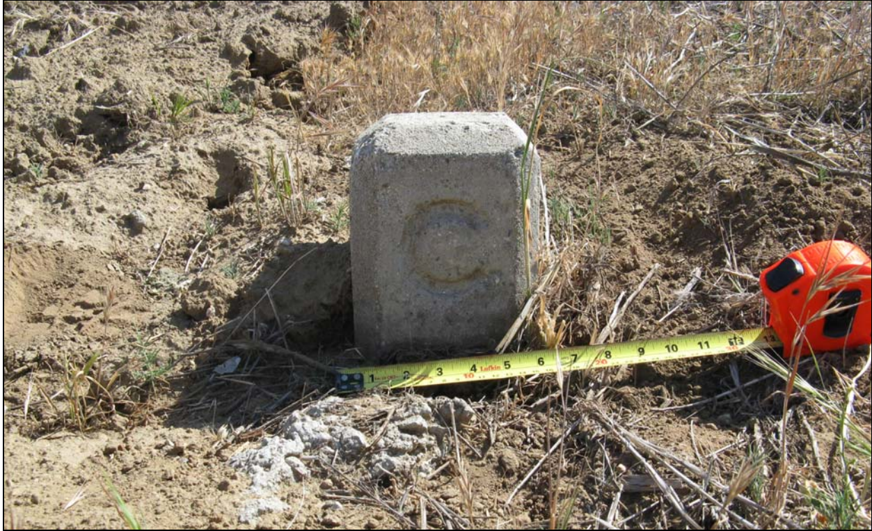
Figure 4. A concrete C monument found along the abandoned curve (photograph taken May 9, 2012, view to the northeast). Note this monument was likely placed at this location in the 1910s.
