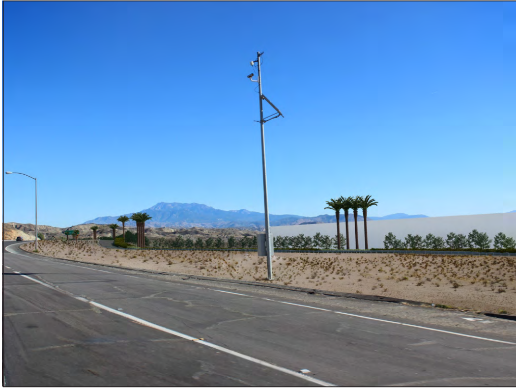
VIEW 7: Looking southeast heading eastbound from SR-60 vegetation at installation.
