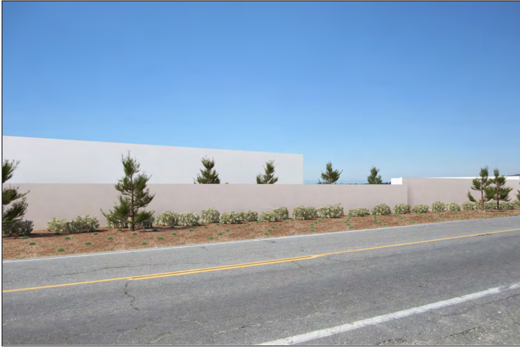
VIEW 5: Looking east across Gilman Springs Road at vegetation at installation.
