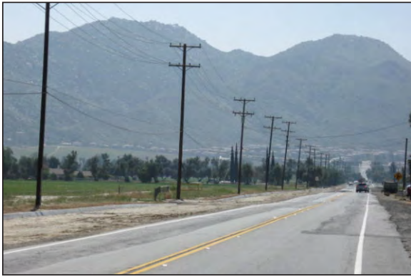
PHOTOGRAPH 1: View looking south along Redlands Boulevard from Eucalyptus Avenue.
