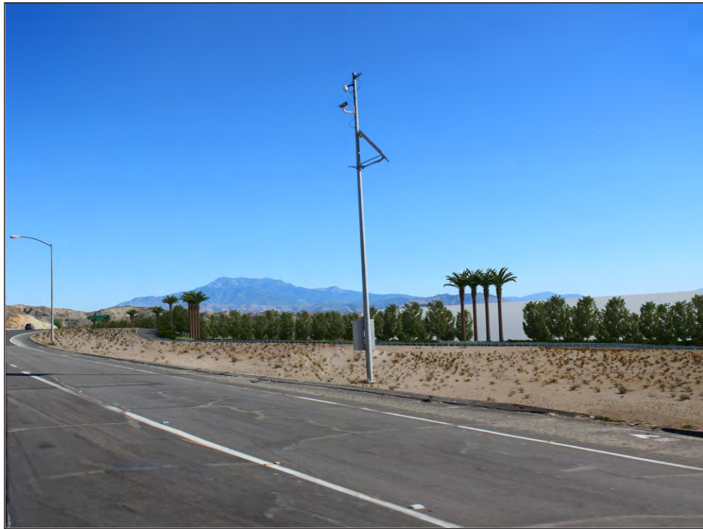
VIEW 7: Looking southeast heading eastbound from SR-60 vegetation at maturity.
