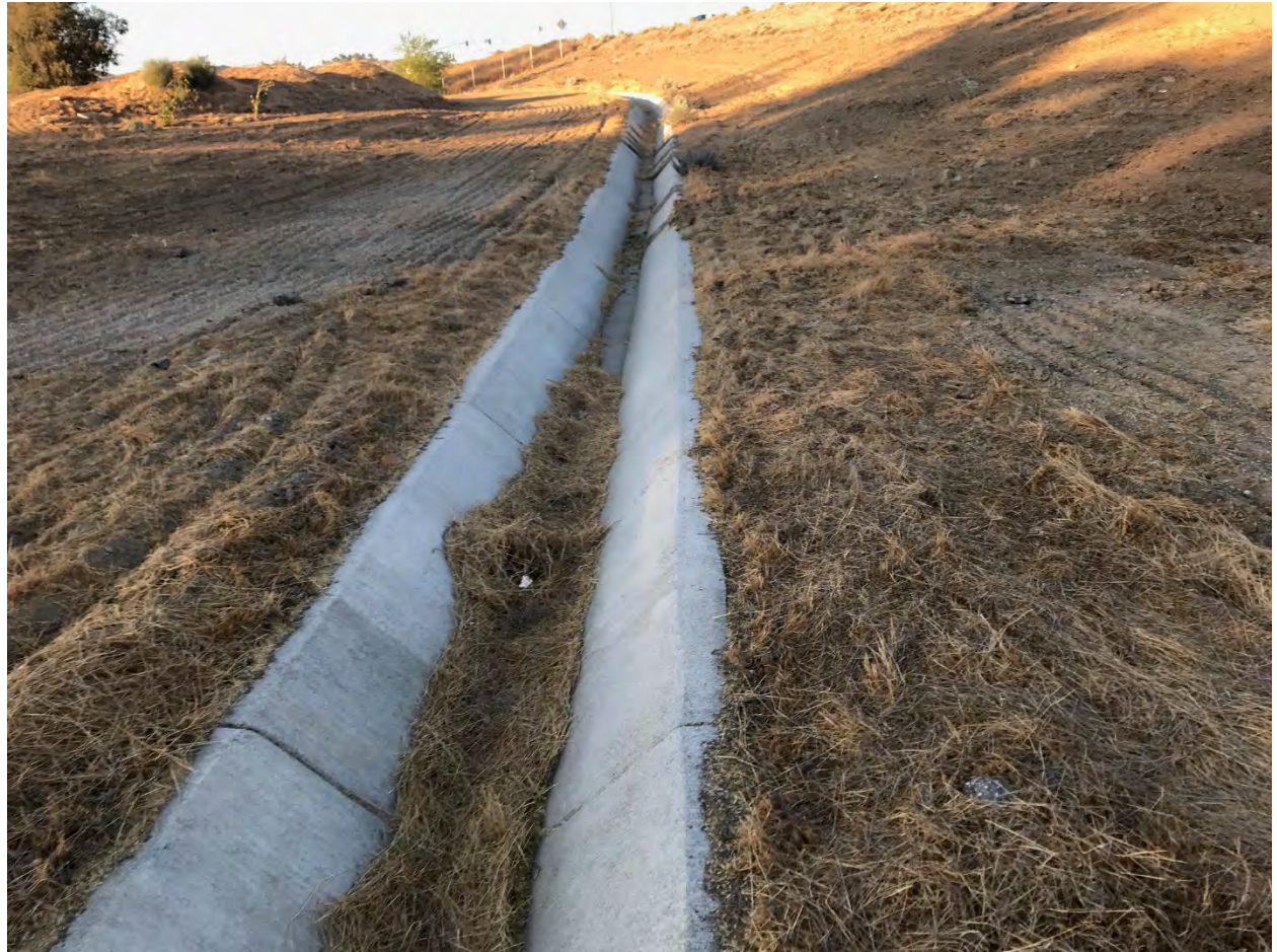
Figure 6 Picture 5 View North
