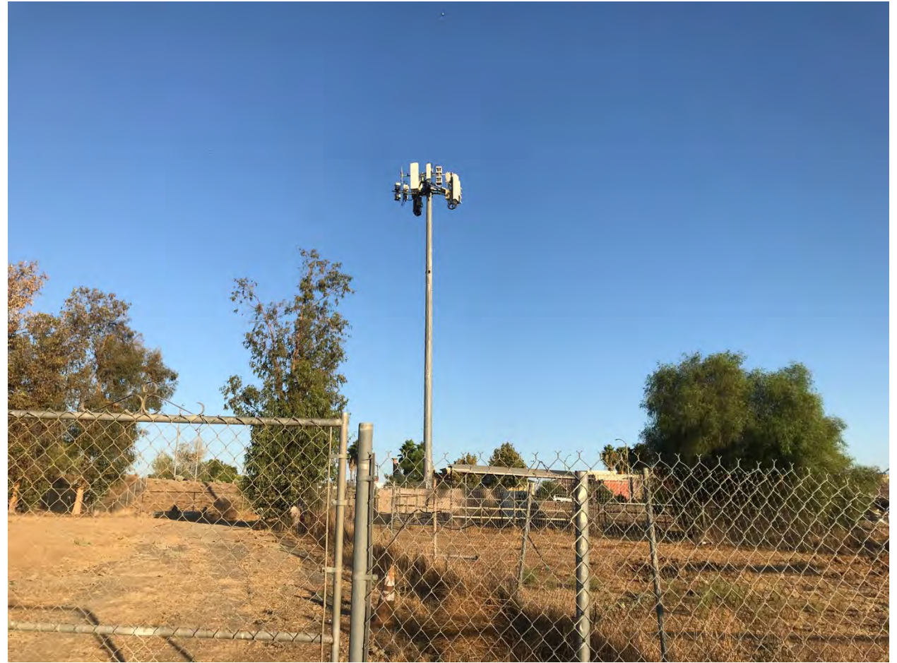
Figure 4 Picture 3 View East
