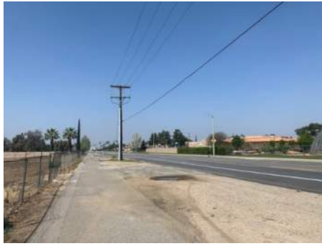
P21- Power Line in the Northwestern Corner of Project Site along Iris Ave.
